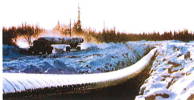
Fig. 7: Pipe laying in Russia – alloying with niobium is essential for pipelines in a cold climate
